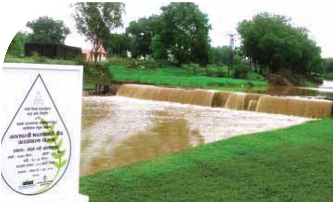
One of the check dams : First rainy season after desilting.
