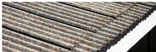
Corrugated asbestos cement sheet as roofing material for roofs of Gaushala is most preferred.
