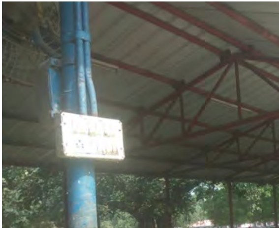
Well insulated electrical switch board and fittings mounted on a pillar on a pillar at approximate height of 6 feet (well beyond the reach of animals).
