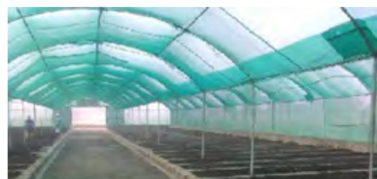
Vermicompost unit with rounded green coloured agro net roof and walls.
