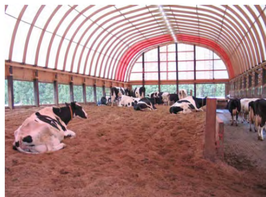
6-8 inches of sand on firm even natural earth. Because of inorganic nature of sand, it absorbs the urine and dung of cow quickly keeping the floors clean, thereby curtailing infections.
