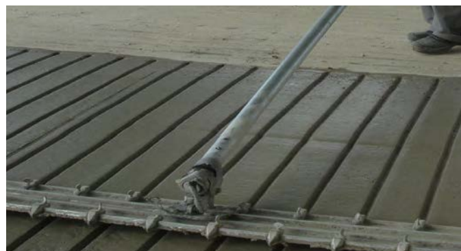
Grooved concrete floor under construction.
