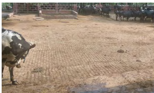
Brick lined floor in cattle shed. Although non slippery nature of floor is favourable, complete cleaning of manure on a brick lined floor is not possible.
