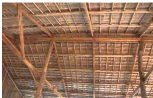
Traditional wood, bamboo and thatch roofs.
