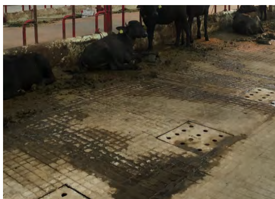
Grooved floor with proper slope towards underground drainage system inside the covered area of a shed.
